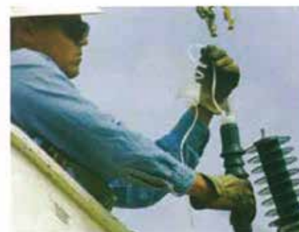
3M™ Coldshrink QT-III Outdoor Terminations
